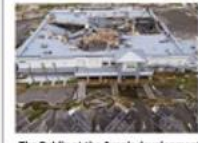
The Publix at the Avenir development was damaged by a tornado spawned by Hurricane Milton on Oct. 10, 2024. GREG LOVETT/PALM BEACH POST
